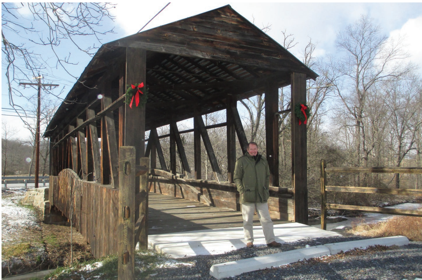
A NEW, OLD BRIDGE: Cecil Cuppett stands at the Cuppett Covered Bridge in New Paris. Cuppett oversaw and financed the reconstruction of the picturesque 1880s bridge in 2015.
